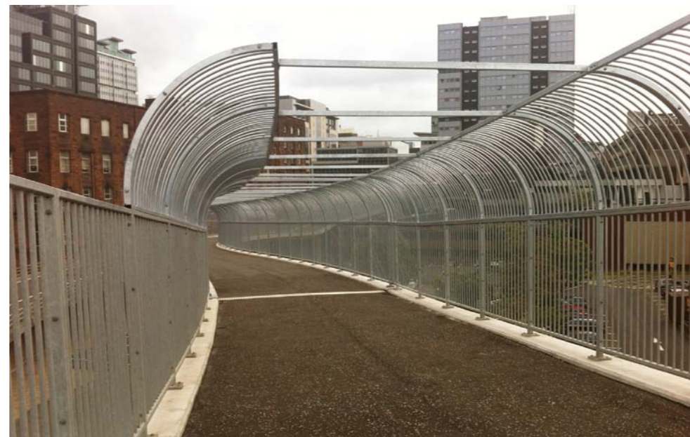
Figure 39: Bridge to Nowhere - a pedestrian bridge across the M8 (Fairhurst 2013)
