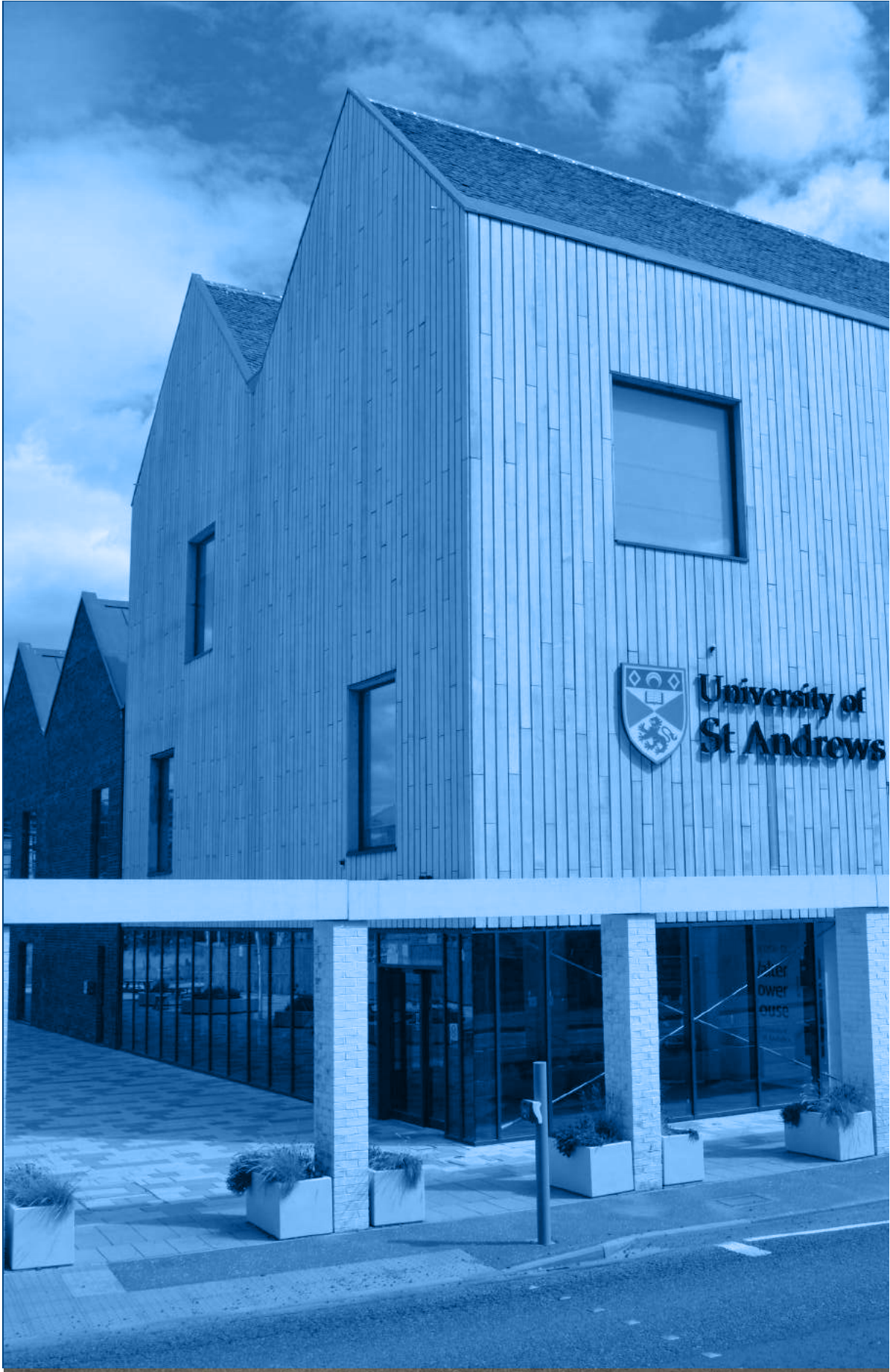
Figure 20. Walter-bower-house, St Andrews University, Eden Campus, Guardbridge, St Andrews.
