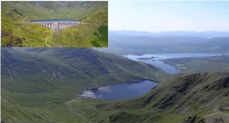
Figure 18 - Cruachan Hydro Pumped Storage Scheme (images from www.visitcruachan.co.uk )
