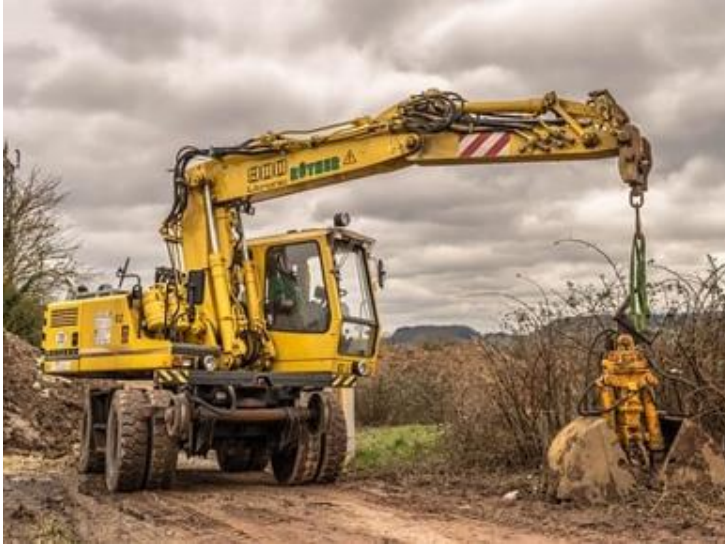
Figure 3 Early-stage construction site
