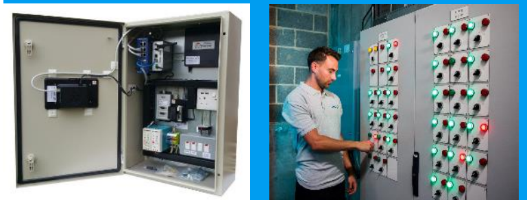
Physical control system units: sizes range from small units in a simple system to a large computer capable of delivering complexities of a large 5G district heating network.
