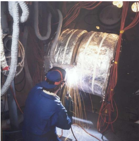
Test Weld in progress in the Hyperbaric chamber
