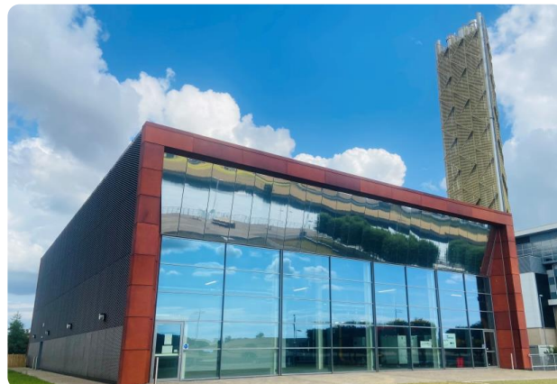
Queens Quay Energy Centre located in Clydebank, Glasgow
