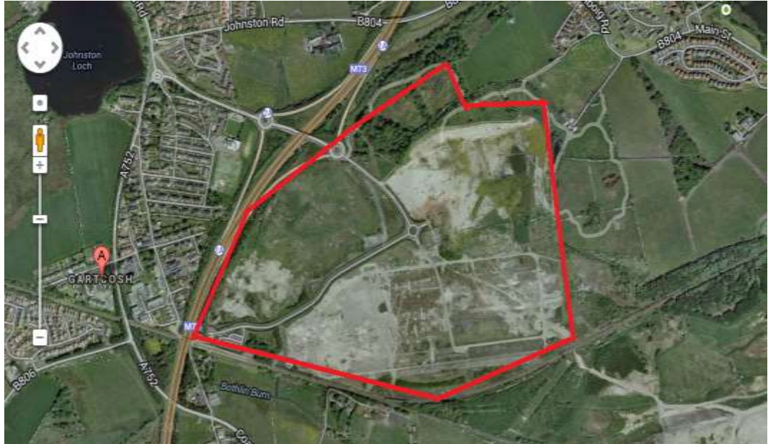
Figure C.5 Aerial view of Gartcosh site
