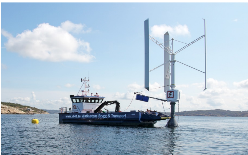
Figure 4 a) Small-scale SeaTwirl S1 rated at 30 kW and b) SeaTwirl S2 turbine concept with underwater spar and ballast. Both figures were taken from the SeaTwirl website [5].
