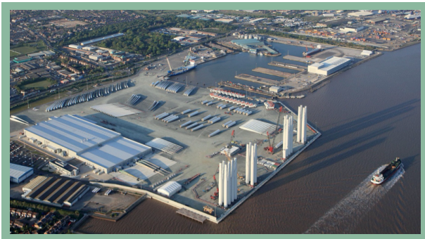
Figure 24 - Green Port Hull is a recent £310million redevelopment Associated British Ports and Siemens of Alexandra Dock to repurpose it for the production of offshore wind turbines.
